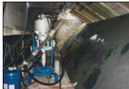
Pitting repaired using ARC 858.
