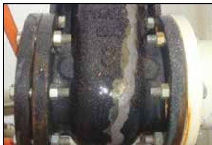
Valve leakage plugged with ARC 5ES.
