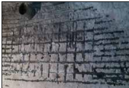
Chest wall after tile removed and blasted.
