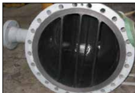
Repaired divider plates.
