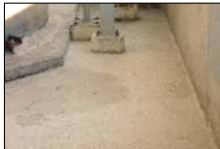
Cleaned and prepared surface.
