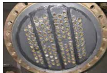
Completed tube sheet.
