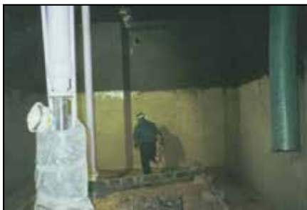
Concrete protected with ARC 791 and ARC 988.
