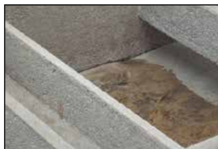
Drained sand filter vessel.
