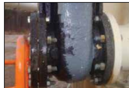
Repaired valve with ARC 5.
