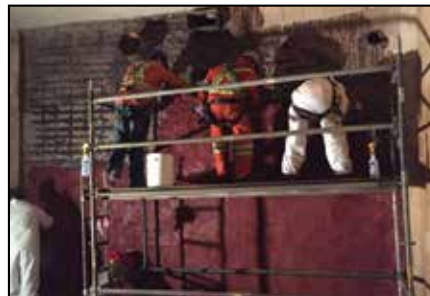
Installing ARC NVE coating.
