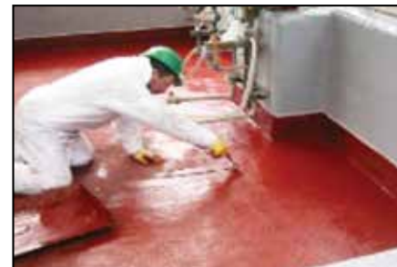
Applying ARC CS4 topcoat.
