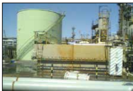
Basin in petrochemical complex.
