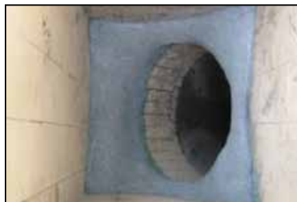
Installation of ARC BX5.
