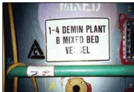
External view of the tank.
