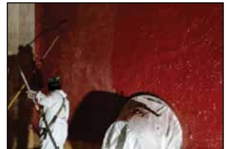
Applying NVE sealer coat.
