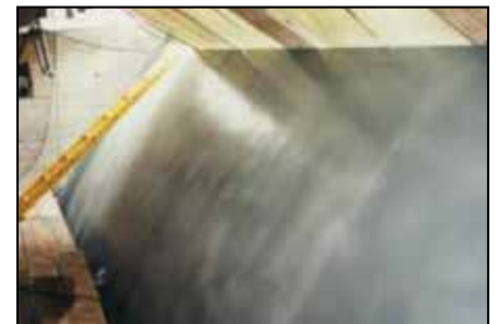
Gate top coated with 2 coats of ARC S2.
