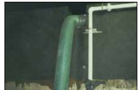
Environmental conditioning required during application.
