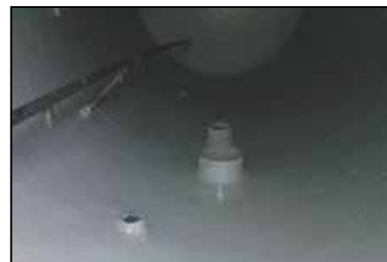
Coated tank internals.
