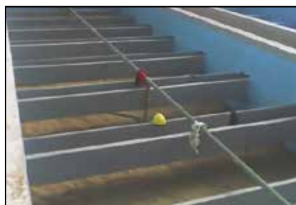
Installing ARC S1PW coating.
