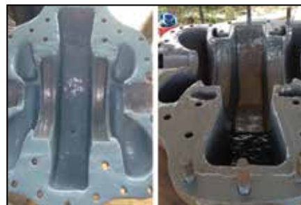
Repair being performed, body and cover.
